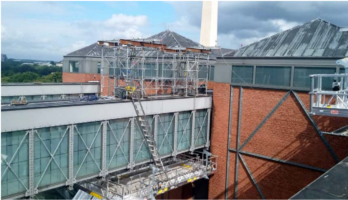
The memorial bridges now have fresh coatings that will protect them for decades.
