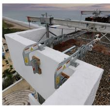
Using a parapet style clamp as a tieback device or lifeline anchor is NOT approved in Canada
