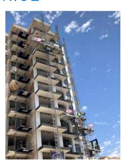
**Mast Compatibility** Personnel & material hoist: EPM 1000 Material hoist: MC 1000 Transport platform: PT 1200
