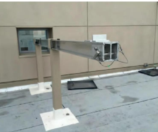
A backfed, fixed outrigger system.
