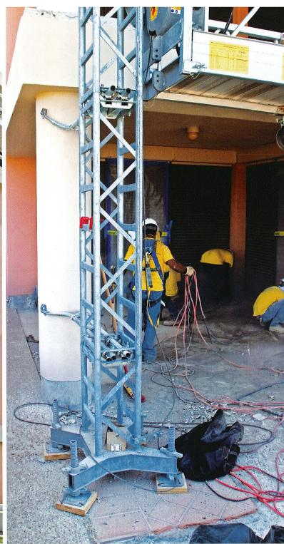
in the future. Also unique is the requirement of a level sensitive electric yoke that prevents the hoists from becoming excessively out of level placing significant loads on the masts and ties.
