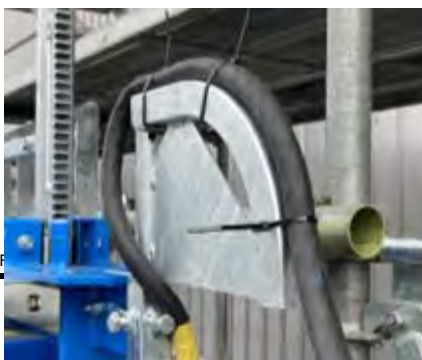
Fitting the cable on hanging bracket
