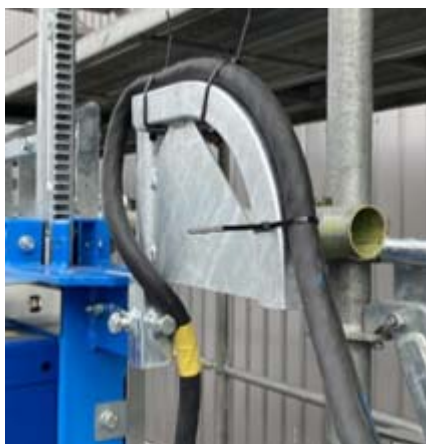
Fitting the cable on hanging bracket
